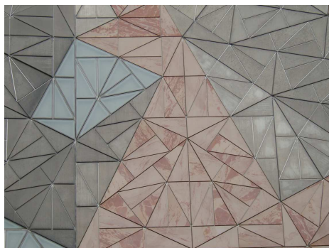
Fig. 35: Detail of a façade at Melbourne's Federation Square featuring a pinwheel tiling. Photography © U. Grimm.
